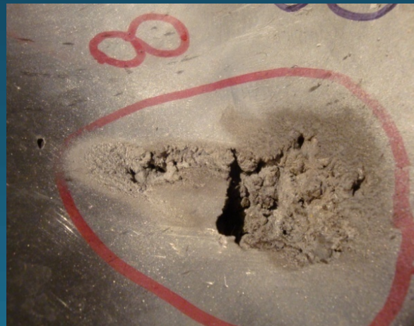
Pelton Bucket damaged regions
